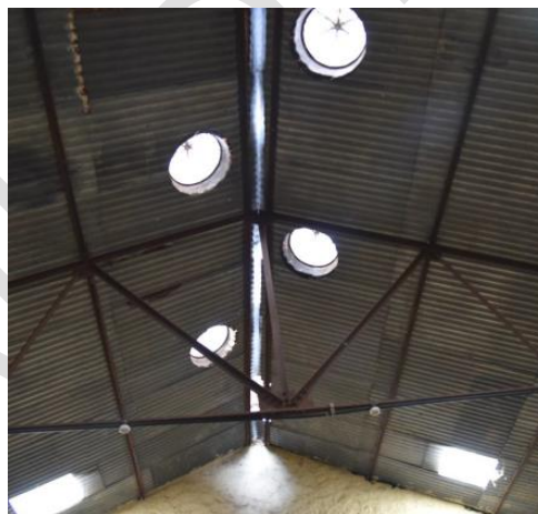
Plate 9: Demonstration of solar lamp, turbo ventilator and asbestos sheet
