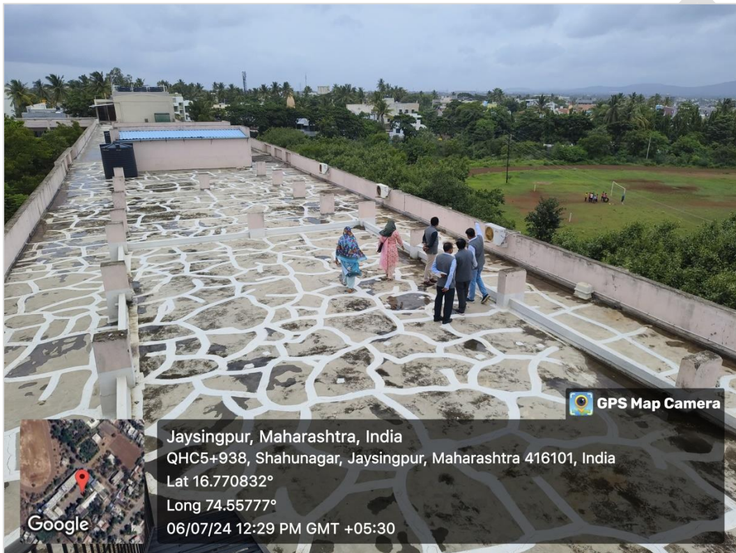
Plate 13: Light colored roof in the premises
